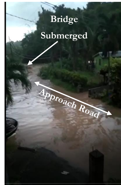
(b) Under Flooding
