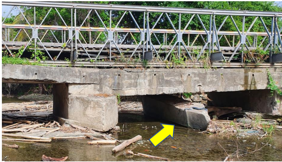
(a) Seamoan Bridge (SB on Fig. 1(a)): Tilted Support
