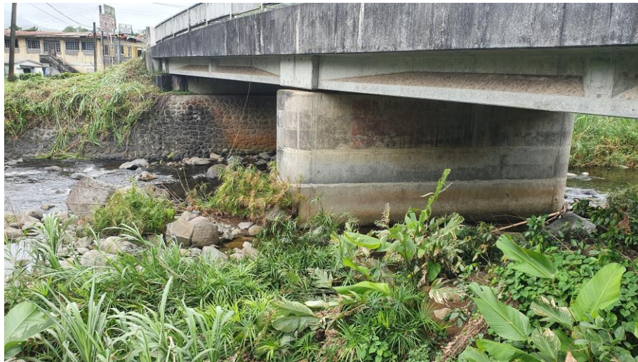
(b) Birch Grove Bridge (BirB on Fig. 1(a)) : Mid-River Support and River Wall Work Well
