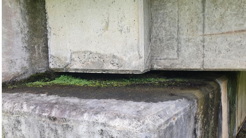
(c) Birch Grove Bridge: Moisture Retention and Plant Growth at Bearing Plinth
